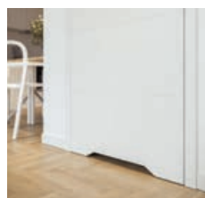
with ventilation undercut
